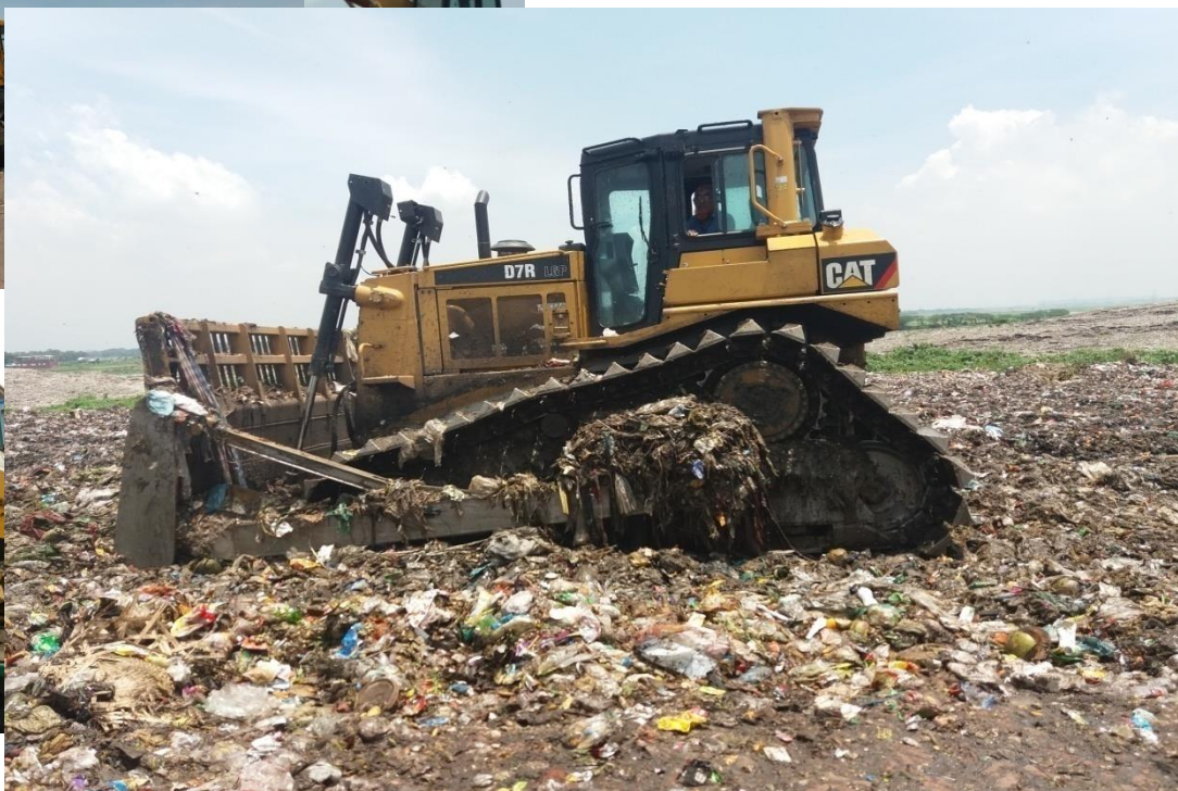
Compaction of waste by chain dozer at Aminbazar landfill
